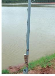
Piezometer being installed in red mud pond area
